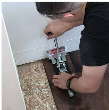
Tighten boards close to walls.
